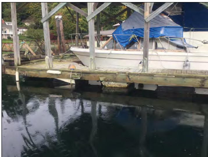
Photo: 3 Old dock with plastic casing falling off styrofoam floats. ( Date Taken: October-12-17 11:40:45 AM, Latitude: 49°38'4.42", Longitude: -124°2'17.82" )
