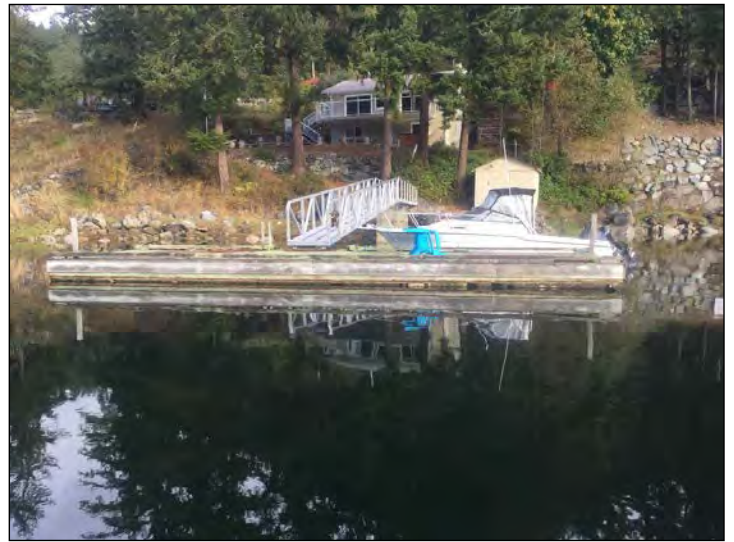
Photo: 20 North shore of Gunboat Bay. Typical wood dock with styrofoam floats. ( Latitude: 49°37'43.55", Longitude: -124°0'17.46", Date Taken: October-11-17 9:35:55 AM )
